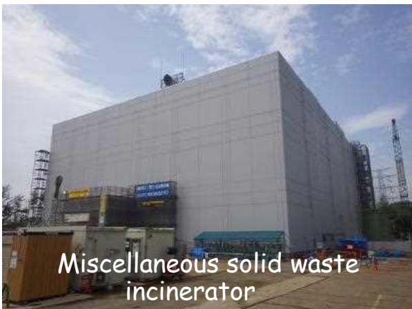
Rubble storage facility
