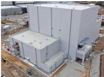
Additional miscellaneous solid waste incineration facility (completed in Mar. 2022)
