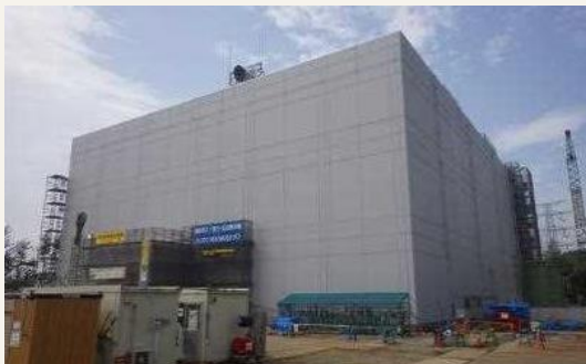
Miscellaneous solid waste incineration facility
