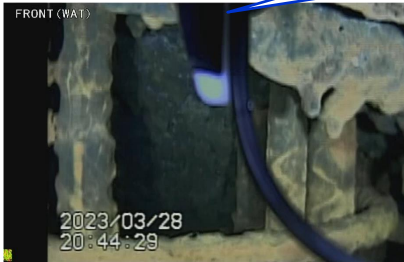
Photo 1: Concrete remains seen from the pedestal opening
