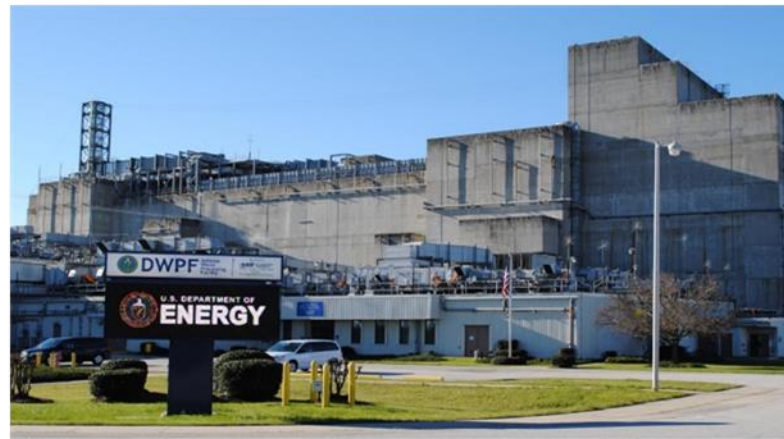
Defense Waste Processing Facility
