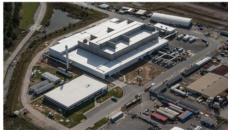
Salt Waste Processing Facility
